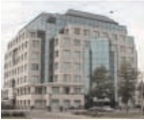
1730 St. Laurent Boulevard Ottawa East Up to 30,038 sq.ft. available for sublease through J.J. Barnicke Limited
