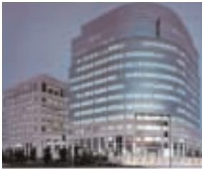
Canada Post Place 655,000 sq. ft. purchased by Canada Post Corporation in Q4 from Standard Life Assurance Company
