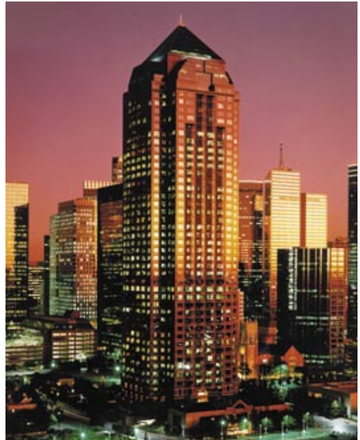
THE TRAMMELL CROW CENTRE, DALLAS
