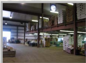
Interior of Warehouse
