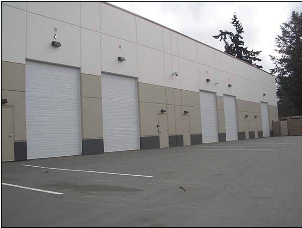
The space has 10' x 14' bay doors and 1 dock-loading door with leveler
