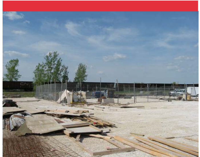
Rear compound potential
