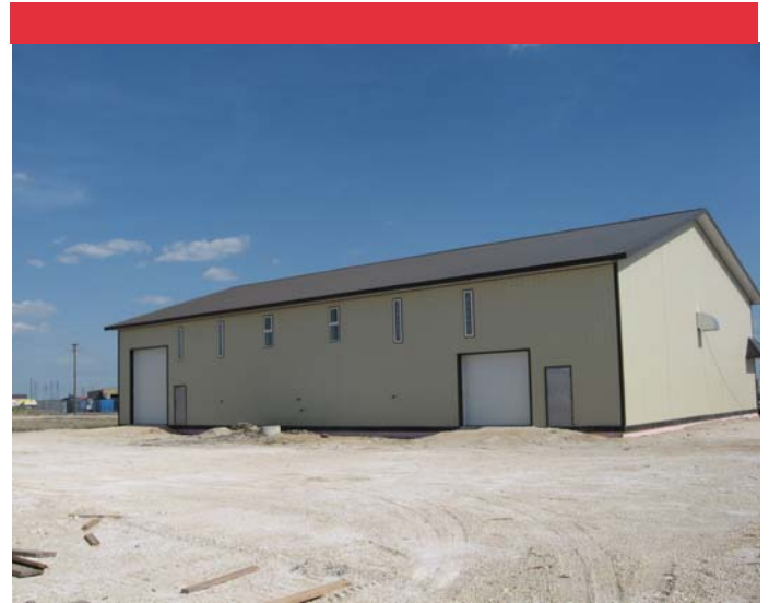
Rear of existing building
